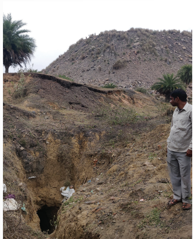
Photo 11: One of numerous treacherous tunnels dug into the ground surrounding the Giridih Open Cast mine, the overburden pile of which is seen in the background. In monsoons these tunnels are notoriously flooded leading to accidents seeing people get buried under the unstable land surface.
